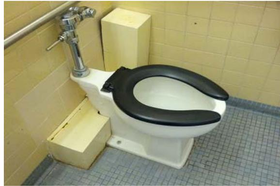
Existing toilets with flow rates of 3.5 gallon per flush or greater will be replaced with high-efficiency toilets.
