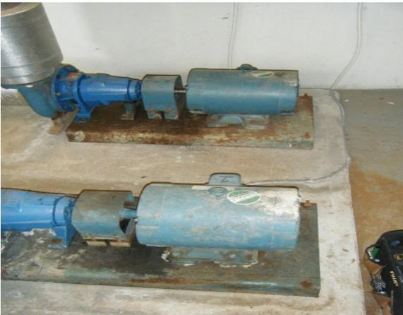
Existing space heating pumps will receive new motors and Variable Speed Drives.
