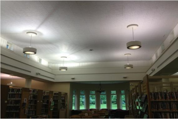
New light fixtures, such as the direct/indirect lighting proposed for the Library will dramatically improve light distribution while providing substantial energy savings.
