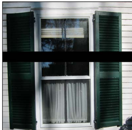
2/2 double hung sash with exterior storm
