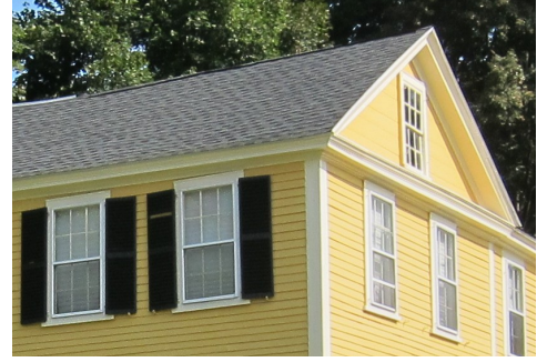
Window casings, corner board, cornice
