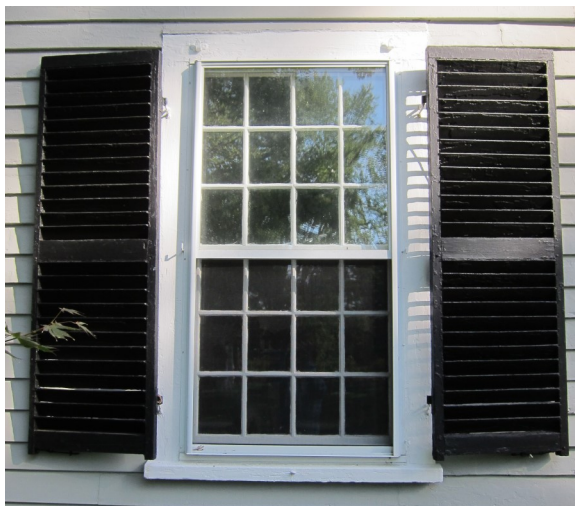
12/12 double hung sash with exterior storm
