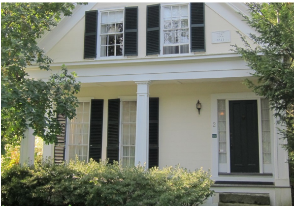
Full length wood louvered shutters flank windows
