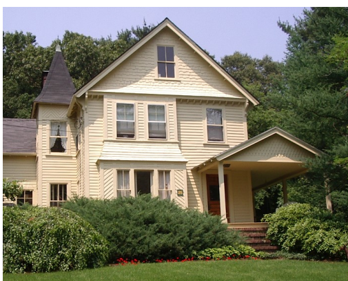
Patterned shingles and clapboards
