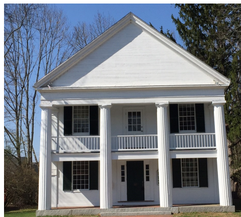
Wood flushboard siding in gable peak
