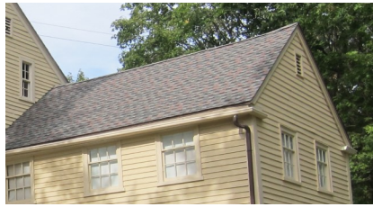
Asphalt shingle roof
