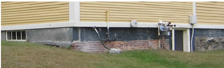
Mixture of brick, stone and granite foundation
