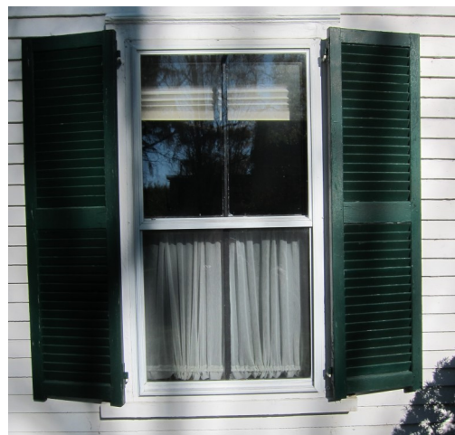
2/2 double hung sash with exterior storm
