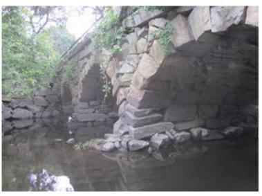
built in 1848. I find this surprising because the dry laid stone construction is very primitive for a time when water resistant mortar materials were commonly available.
