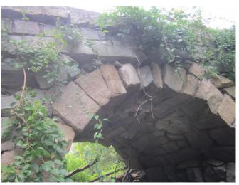
or chinkers have fallen out, revealing cavities within the arch and sidewall construction.
