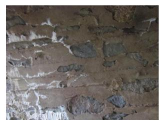
3. The wedge-shaped "valleys" between the arches were filled in with solidly mortared stone rubble to provide a flat surface that would not collect water. The far ends of the arch runs were squared off with fully mortared stone rubble to create buttresses that would press against the earth at each abutment to prevent spreading of the arches.
