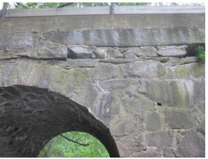
• There are other scattered areas where the stonework has become loose or shifted, particularly at the end approaches, which were dry-laid and then tuck pointed with mortar.
