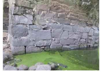
cutting and repointing. These surfaces include the wing walls, parapet walls, and the ends of the arches and "wedge" sections.
