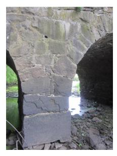
2. Arched wooden forms were then constructed between the piers to support the construction of fully mortar bedded single wythe stone arches rising approximately 5-feet off of the piers. The board form lines can be seen on the intrados of each arch, where the bedding mortar was squeezed out from between the arch stones onto the forms and then hardened.
