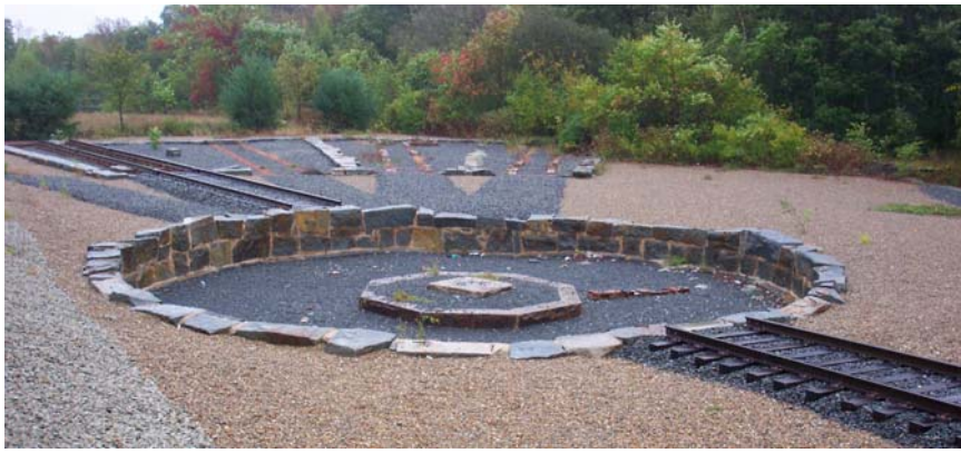
Figure 23a and b. Turntable and enginehouse foundations at Whitman Roundhouse Archeological Park, Whitman, Massachusetts, (HWA, 2004).
