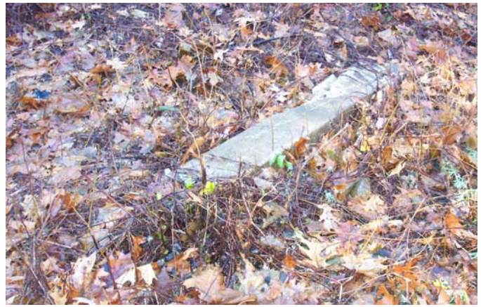
Figure 12. Toppled and broken whistle post, (HWA, 2004).
