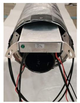
10) Fish the Light Wire inside the Pole via the Hole provided.
