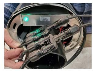
5) Disconnect the Black Connectors by Pinching it using your Hands or a Flat Head Screwdriver.
