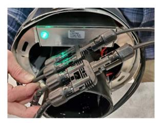
12) Push the Red Connector and 2 Black Connectors around the Battery Boxes inside the Array.
