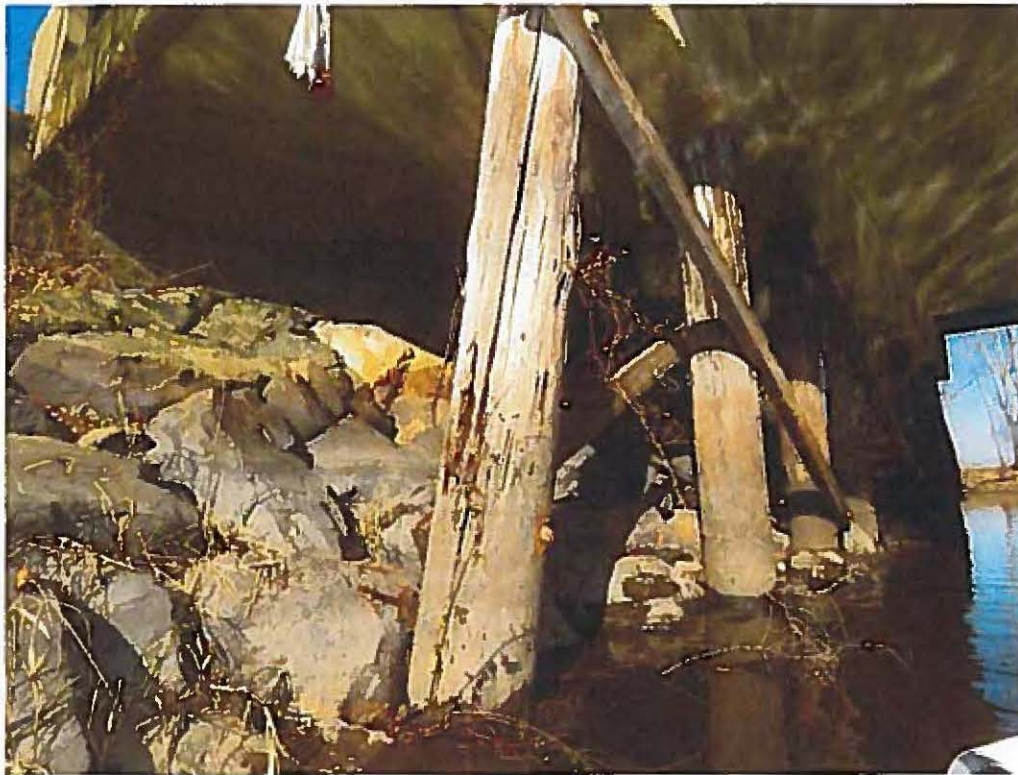
Photo 15: Pile bent #1.
