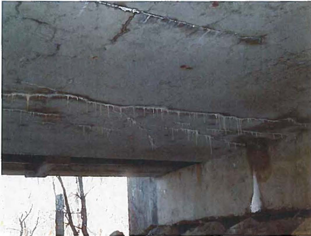
Photo 5: Deterioration to the deck underside in span #6. Northeast corner of the bridge.
