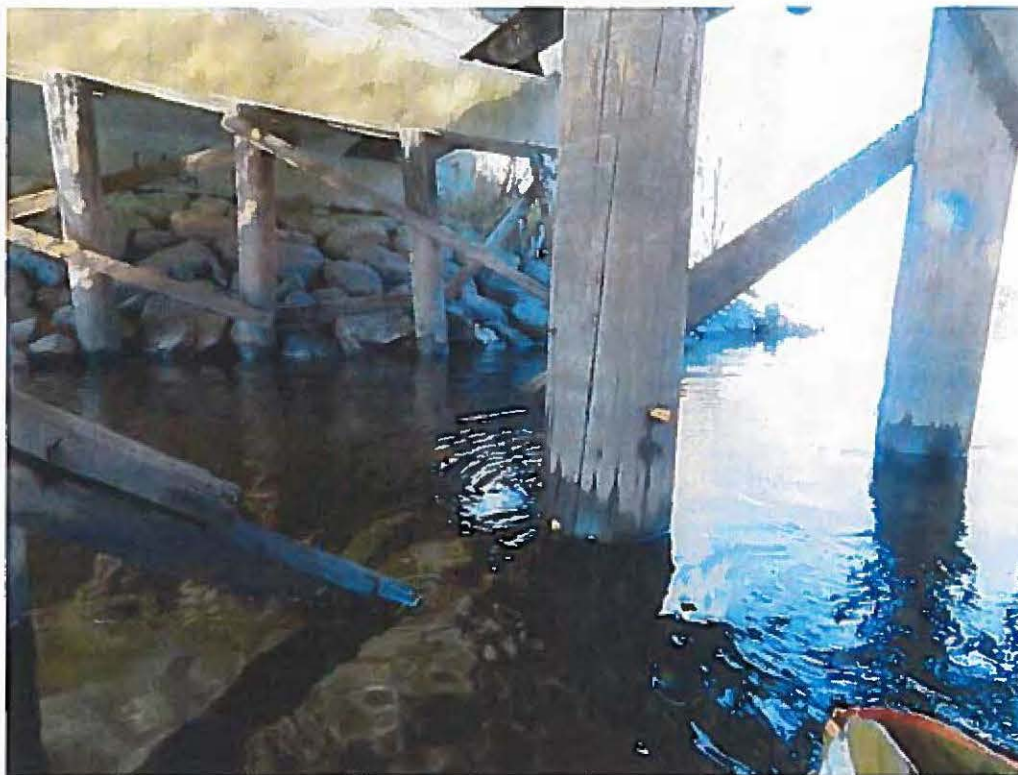
Photo 19: Broken/disconnected diagonal brace on bent #2.
