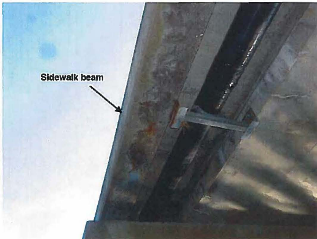
Photo 10: Typical condition of the sidewalk beam.
