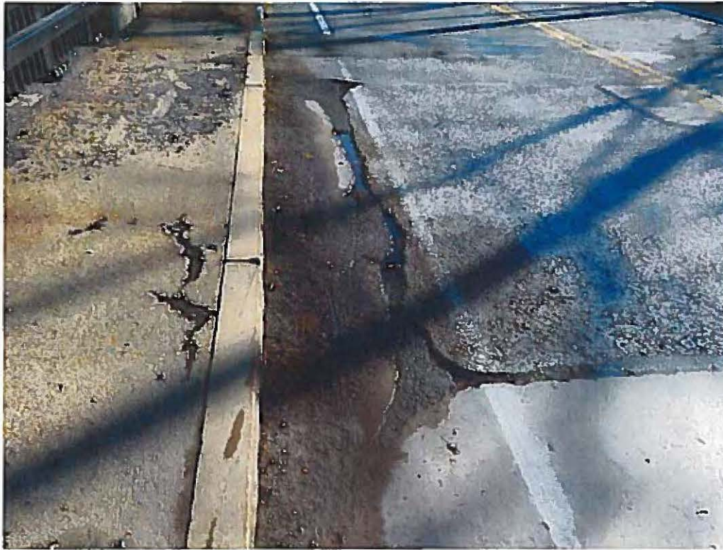
Photo 3: Deterioration at the Northeast corner of the wearing surface.
