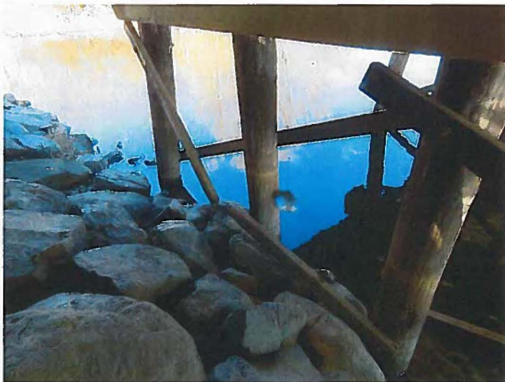
Photo 18: Broken diagonal bracing between piles #6 and #8, bent #1.
