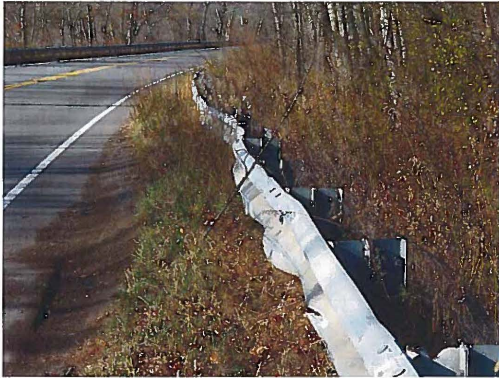
Photo 21: Collision damage to the Northwest approach guardrail.
