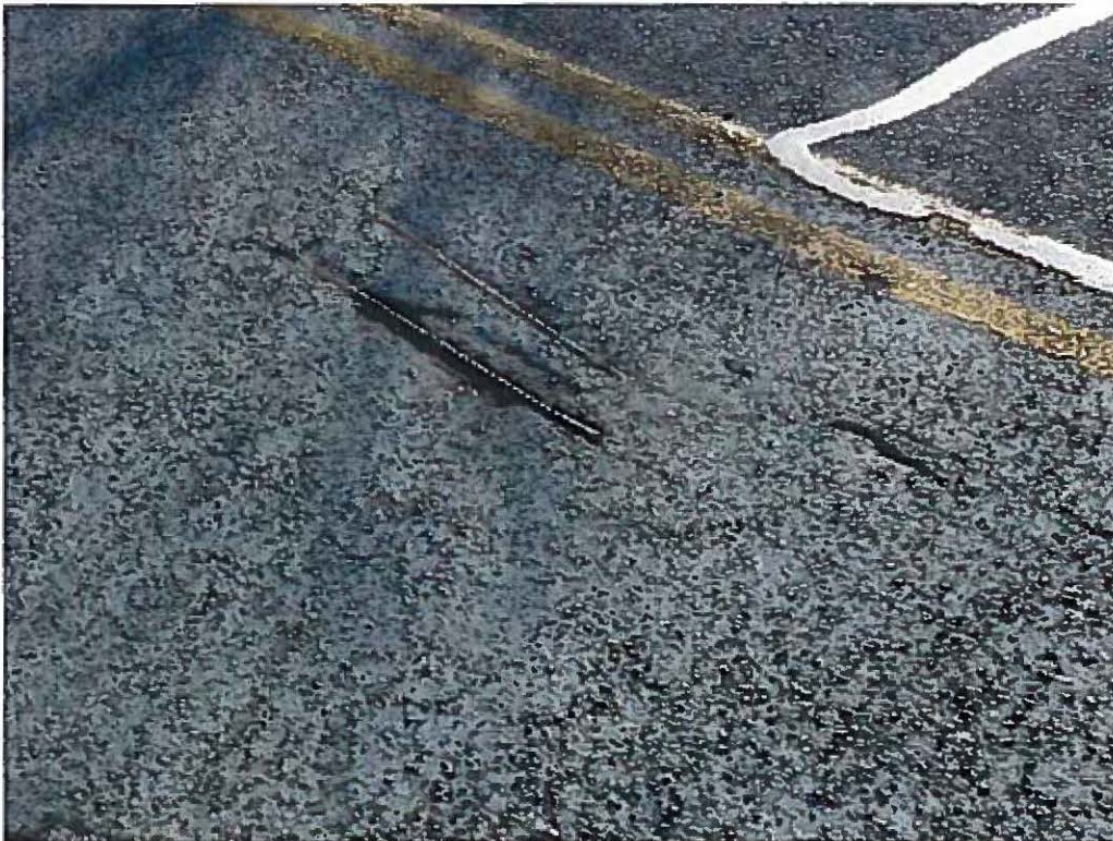
Photo 2: Shallow spalls exposing rebar in the Westbound travel lane.
