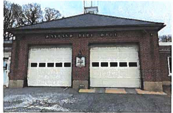
EXISTING APPARATUS BAY ENTRANCE
