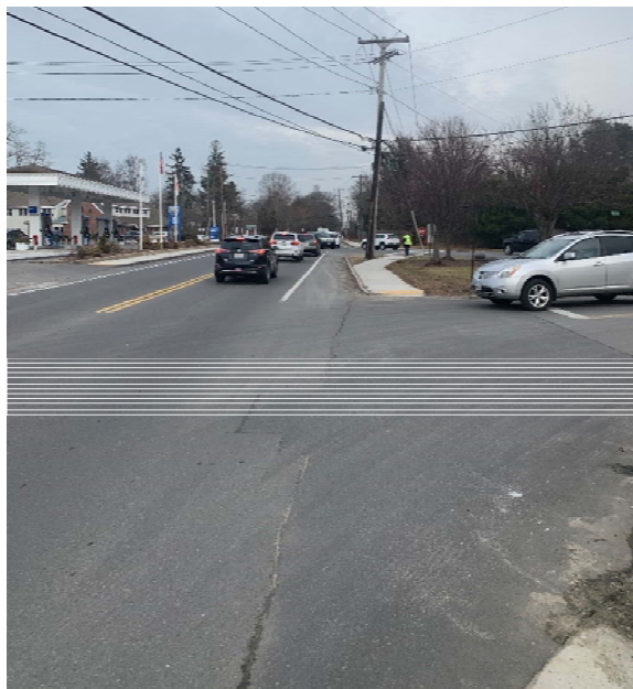
Figure 7: Missing crosswalk across western Old Connecticut Path approach
