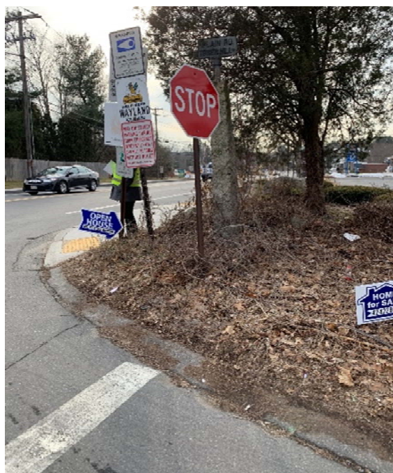
Figure 8: Poor sight distance from Plain Road
