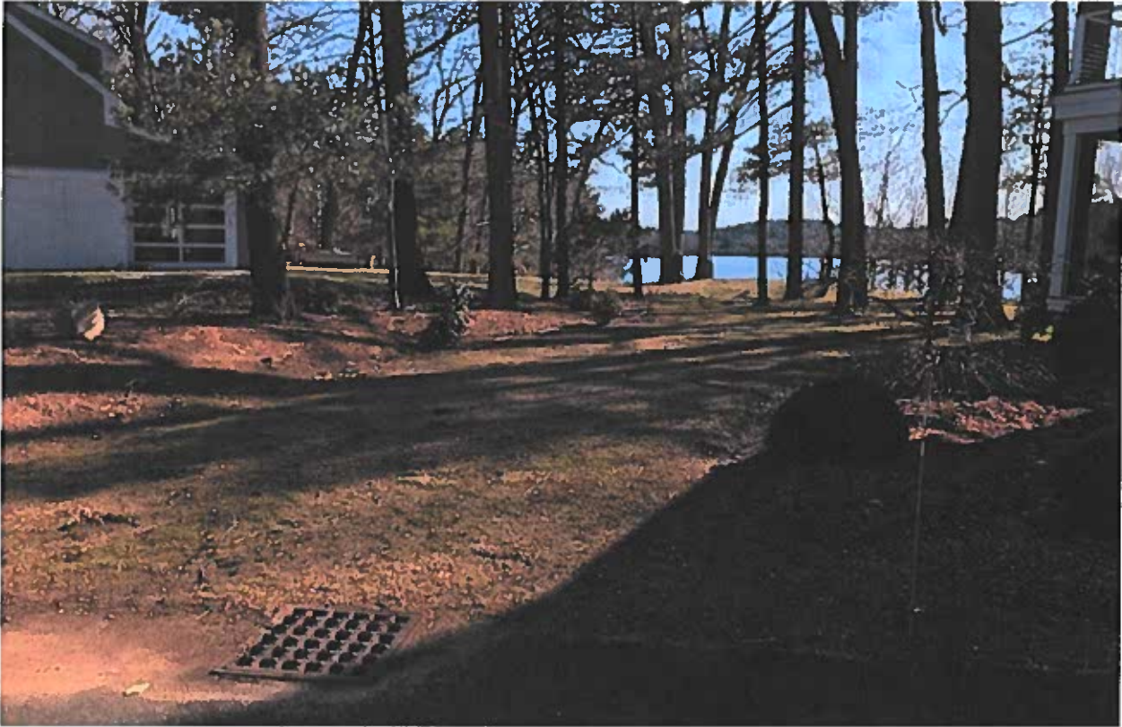
Photo 3: View of Side Yard over Drainage System
