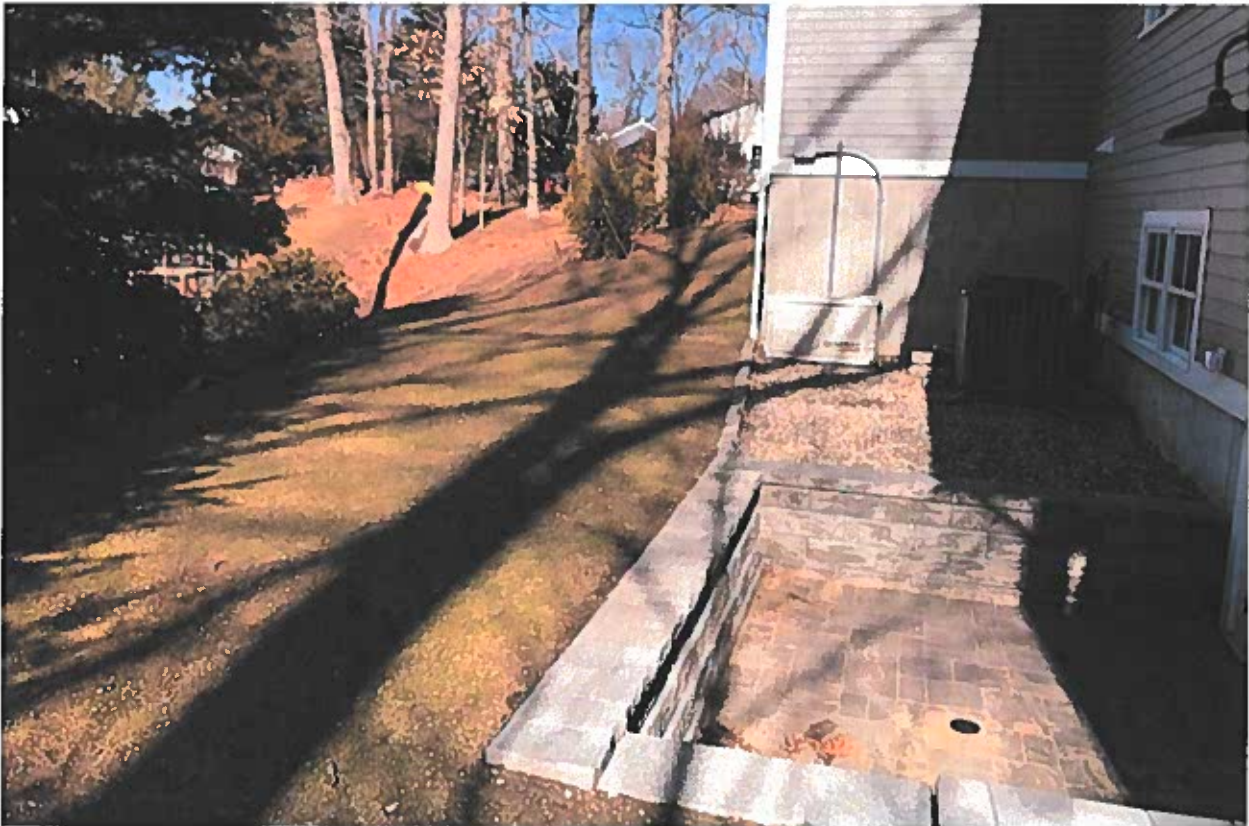
Photo 5: View of Rear Yard – Abutter side
