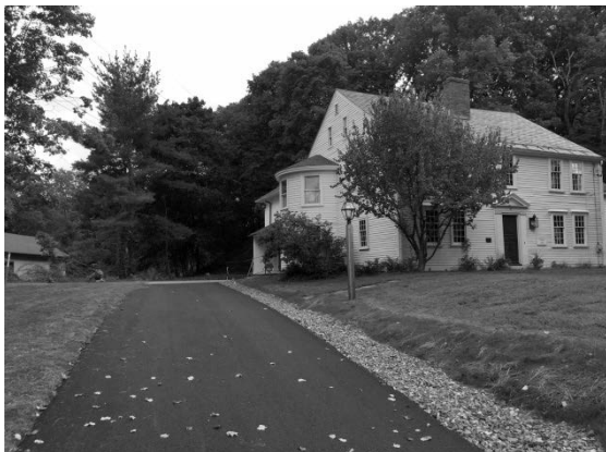
New driveway at Grout-Heard House & Museum
