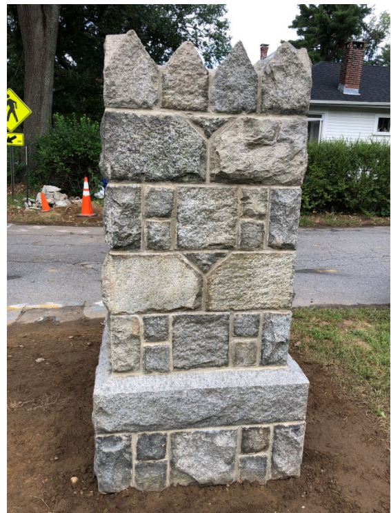
Mansion Inn Pillars at Castle Gate - Reconstructed
