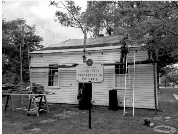
Mellen Law Office Project with new CPA sign
