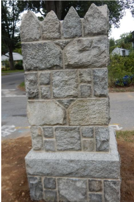
Restored Castlegate Pillar
