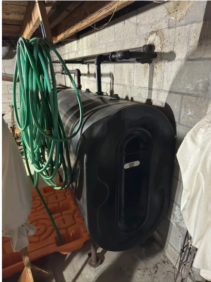
Basement – oil tanks along north wall of main block
