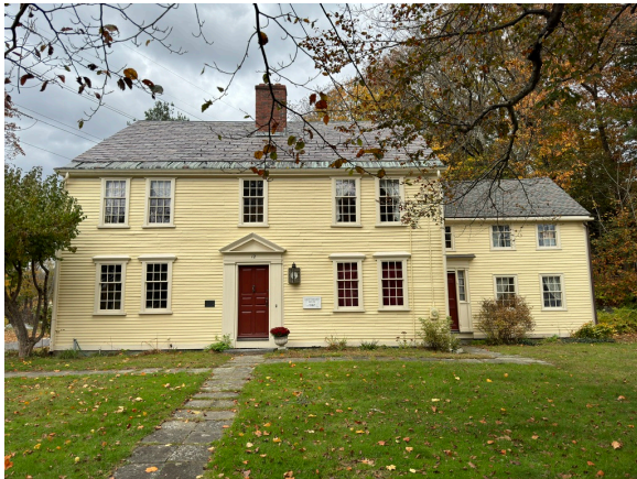
Facade of Grout-Heard House Museum – looking east
