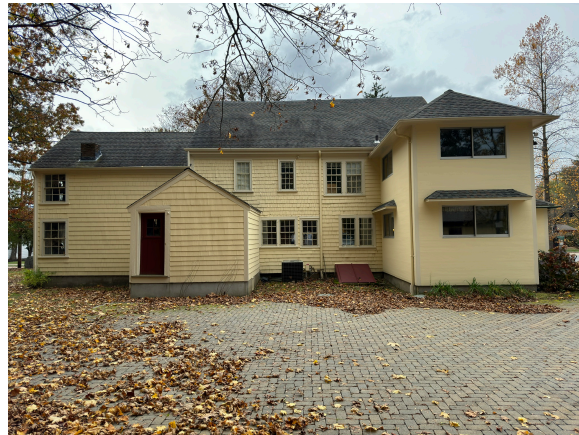
Rear Elevation of GHM – looking west
