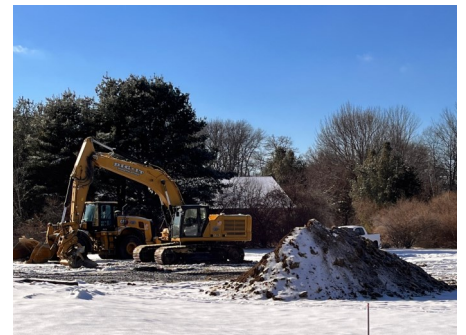
The work begins, January 2024
