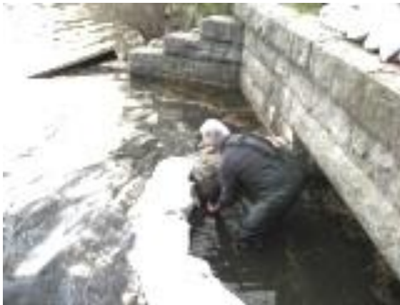
Lowery's Dudley Pond Dam
