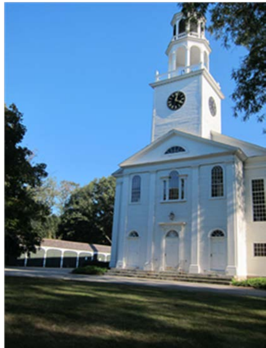
First Parish Church restored windows and Carriage Sheds new wood roof
