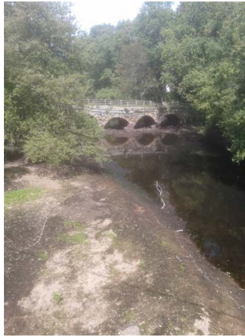
Sudbury River, Old Stone's Bridge adjacent to 246 Stonebridge Road
