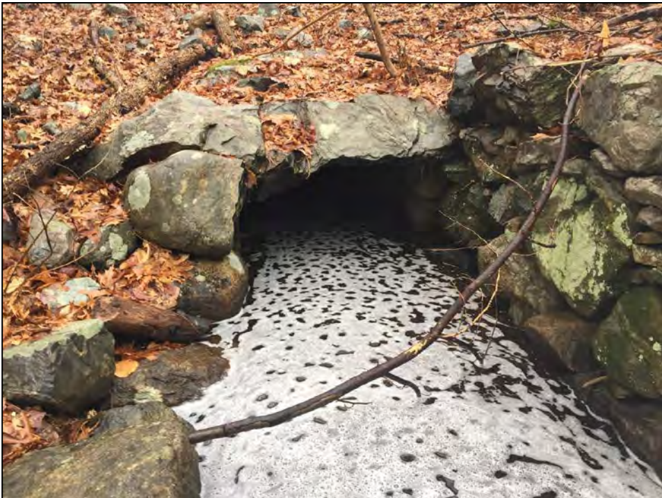
Photo No. 26: Outlet end of the outlet culvert
