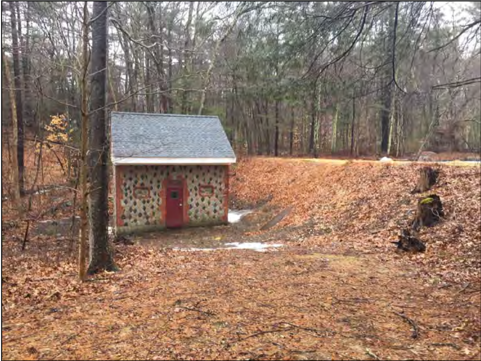
Photo No. 2: Overview of the downstream side of the dam.
