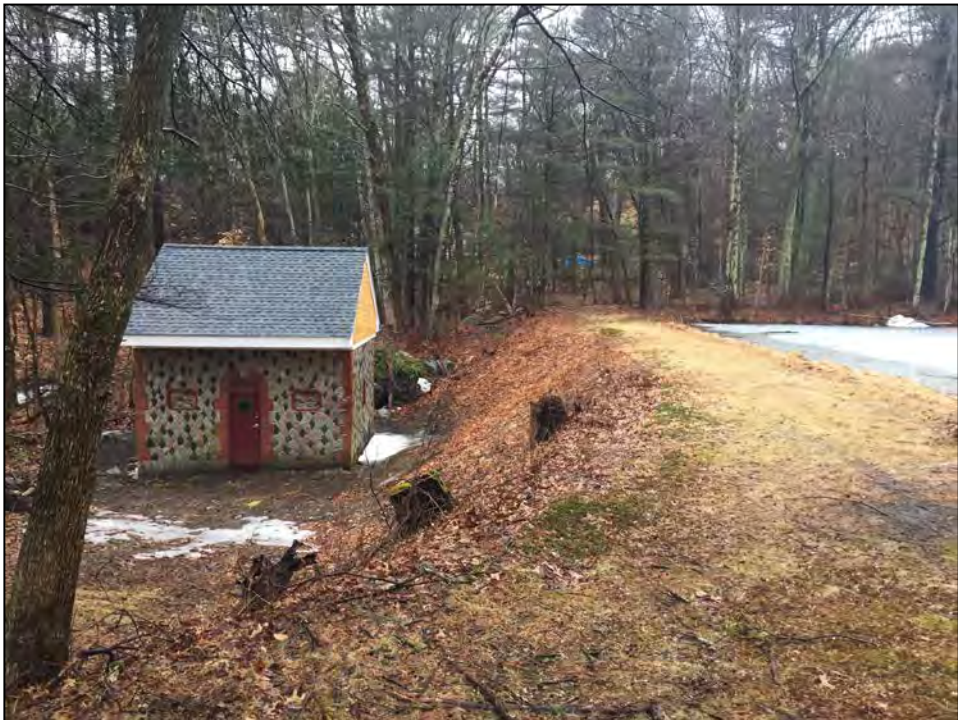
Photo No. 7: Downstream slope from the left abutment looking right.
