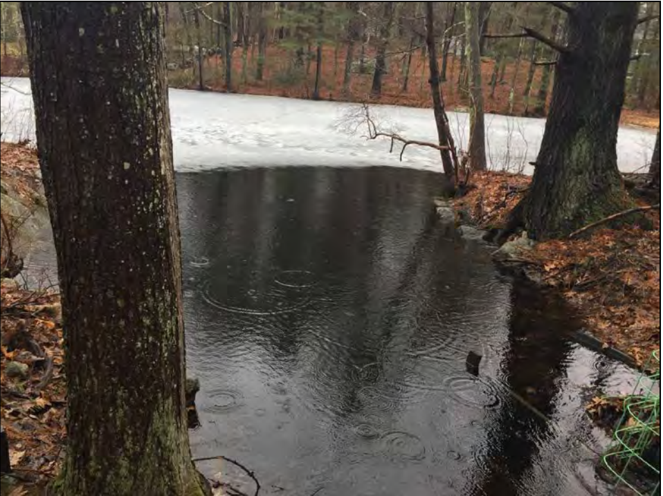
Photo No. 10: Spillway approach from the control section looking upstream.
