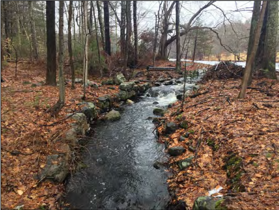
Photo No. 14: Discharge channel of the spillway.
