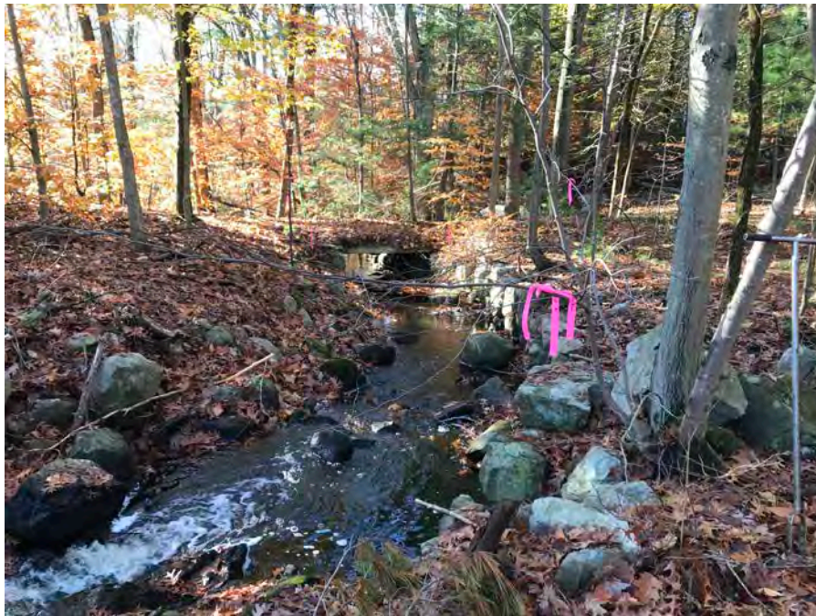
Photo 6: Outlet channel, facing downstream from spillway toward footbridge.
