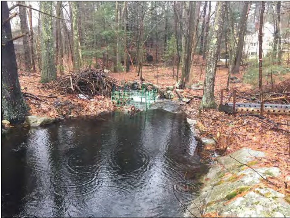
Photo No. 11: Spillway control section from the approach looking downstream. Note apparent bedrock outcrop in picture foreground.
