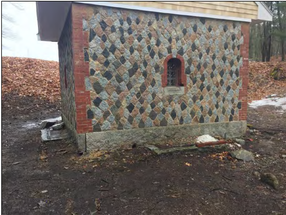
Photo No. 24: Downstream wall of the gatehouse superstructure.
