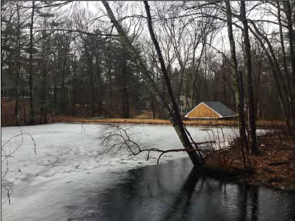
Photo No. 4: Overview of the upstream face of the dam from the spillway approach looking downstream and left..
