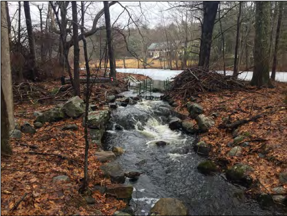
Photo No. 13: Discharge channel of the spillway.
