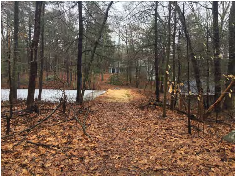
Photo No. 5: Crest of the dam from the stone culvert looking left.
