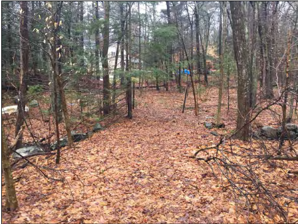
Photo No. 6: Crest of the dam looking right.
