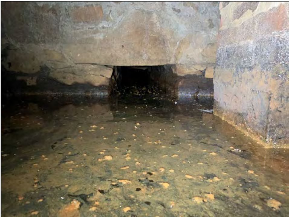
Photo No. 22: Outlet culvert.
