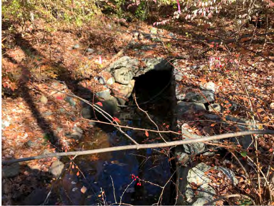
Photo 7: Walled outlet channel downstream of dam, located between flags R-12 and R-15.
