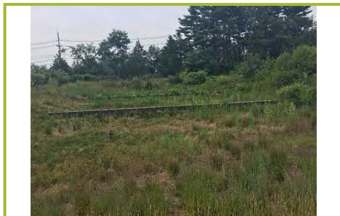
Photograph #28: Wastewater treatment ponds.
