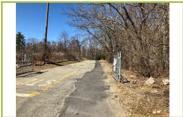
Photograph #37: Eastern abutting access road toward the Wayland Transfer Station.
