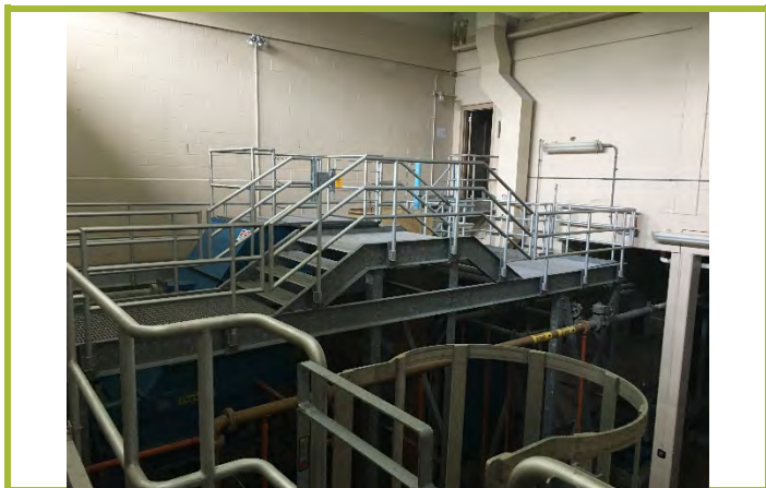
Photograph #13: Area open to basement.
