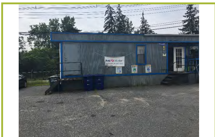
Photograph #29: Office trailer, facing south.
