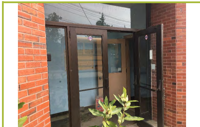
Photograph #2: Main site building entrance.
