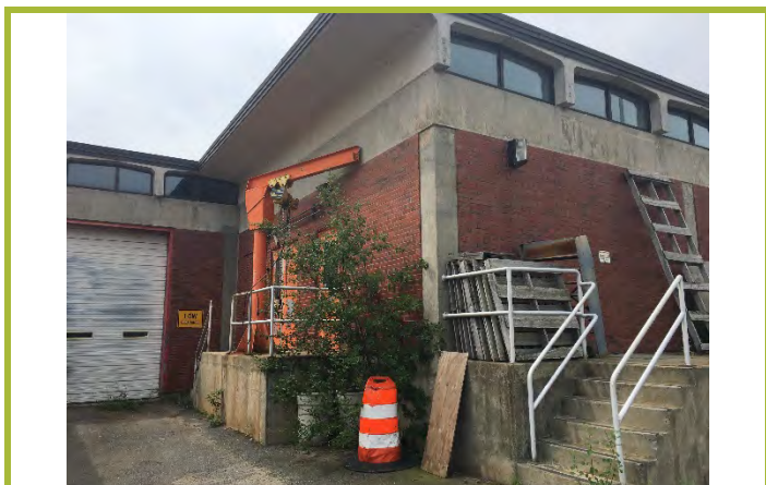
Photograph #3: Northeastern exterior corner of the site building.
