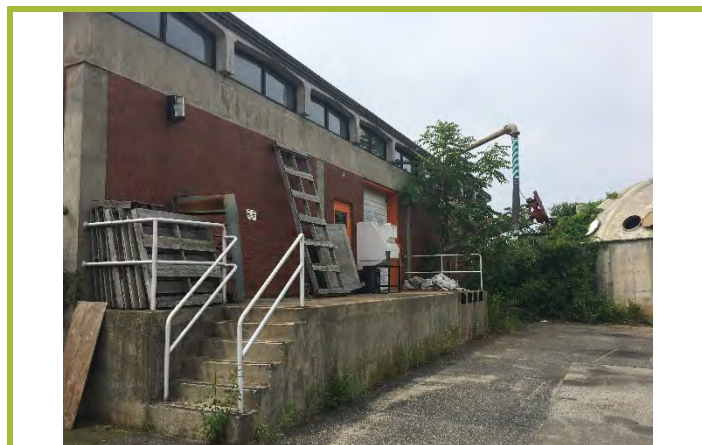
Photograph #4: Northern exterior wall of site building.
