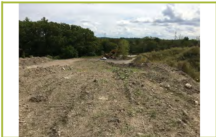
Photograph #31: Top of 32,000 cubic yard stockpile, facing southeast.
