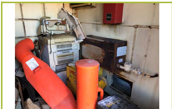
Photograph #25: Material storage and flammable storage cabinet within the northern portion of the trailer.
