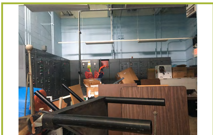
Photograph #11: Control room filled with various school furniture.
