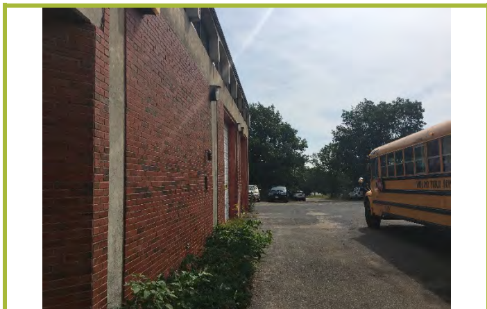
Photograph #1: Southern exterior wall of site building, facing east.
