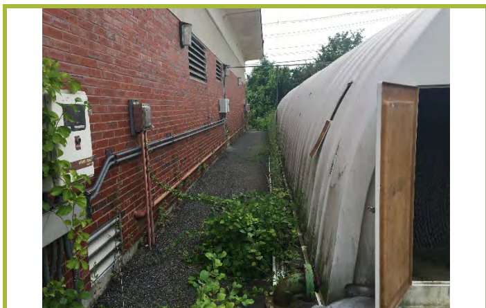
Photograph #27: Western exterior wall of site building and exterior treatment structure.
