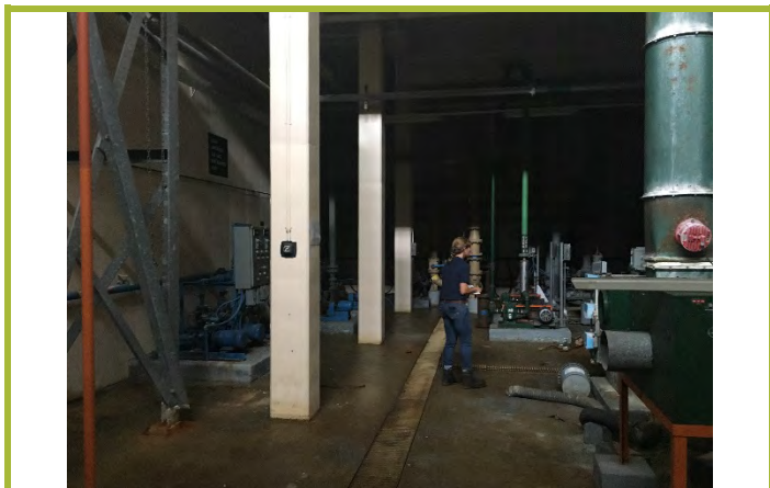
Photograph #19: Basement machine area and floor drains.
