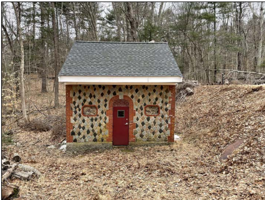
Photo No. 18.: Left side of the gatehouse.
