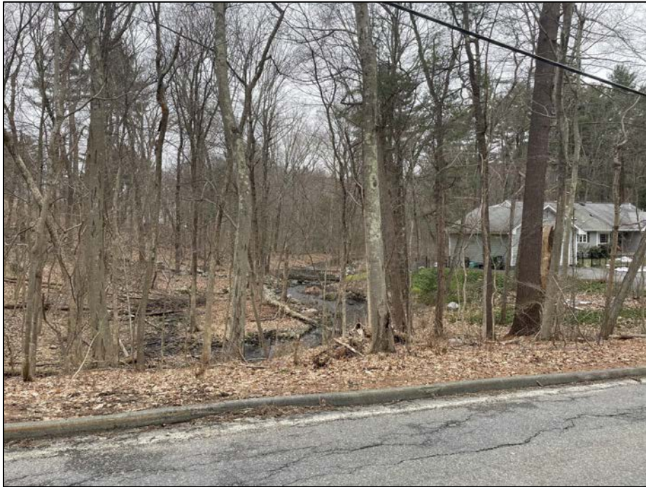
Photo No. 23.: Downstream channel from Woodbridge Road looking downstream.
