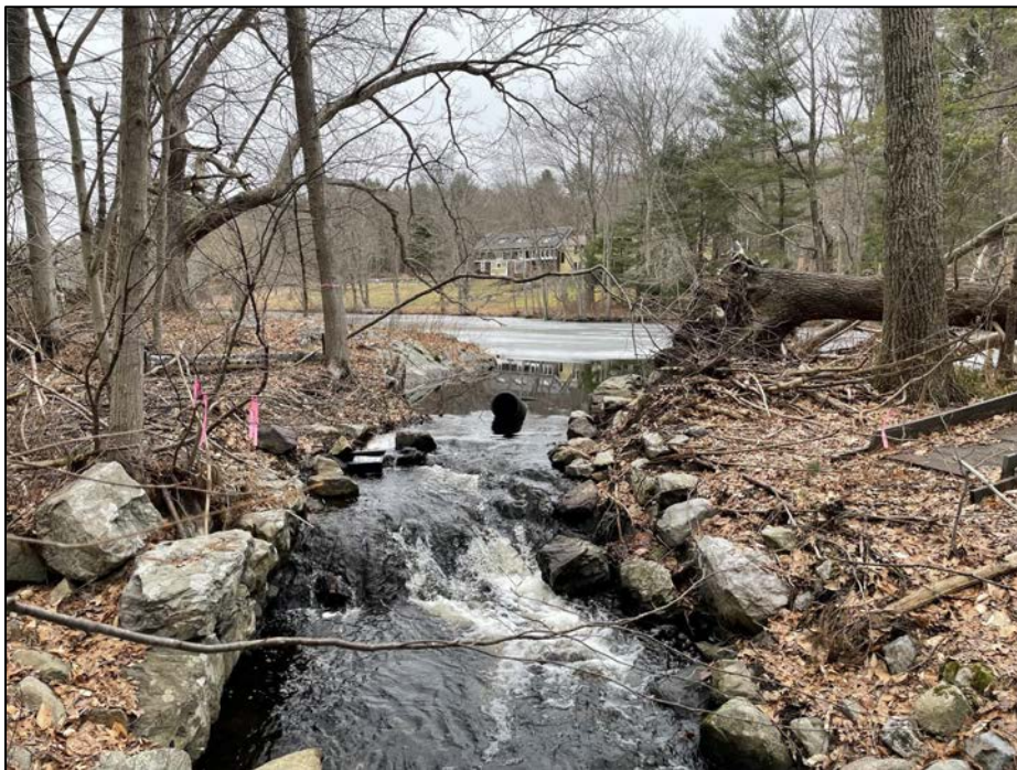
Photo No. 14.: Spillway control section from the discharge channel looking upstream.
