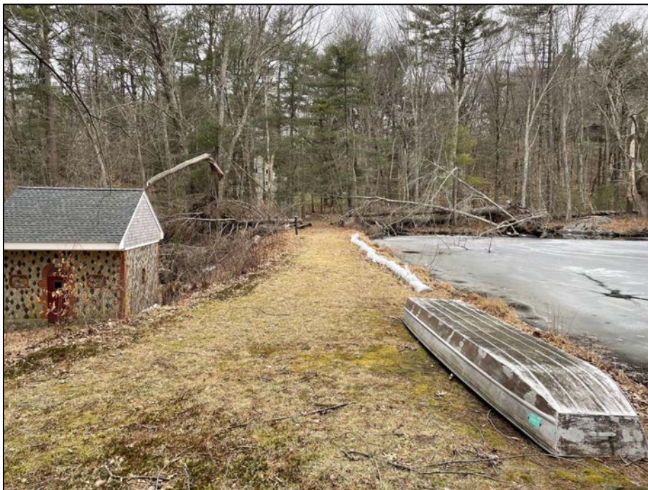
Photo No. 6.: Crest of the dam from the left abutment looking right.
