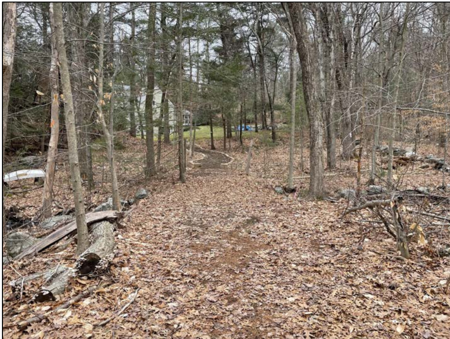
Photo No. 8.: Crest of the dam from near 1+40 looking right.
