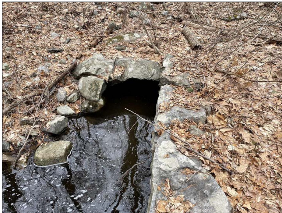
Photo No. 20.: Downstream end of the stone culvert looking upstream.
