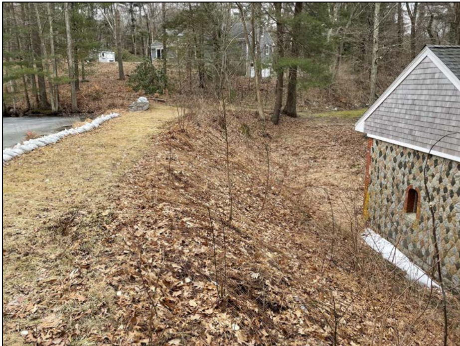
Photo No. 10.: Downstream side of the dam from near 1+00 looking left.
