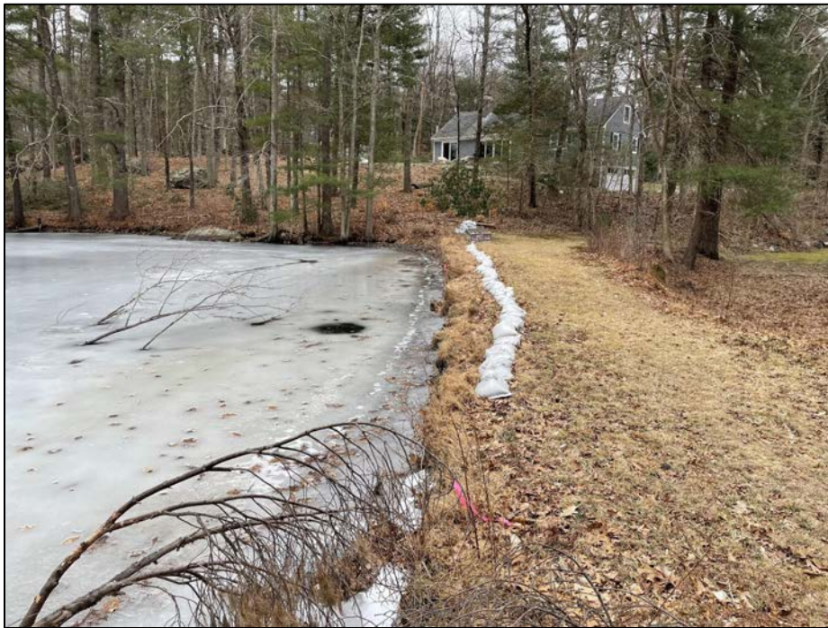
Photo No. 5.: Upstream slope from near 1+30 looking left.
