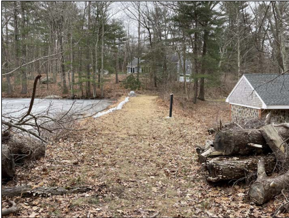
Photo No. 7.: Crest of the dam from near 1+40 looking left.
