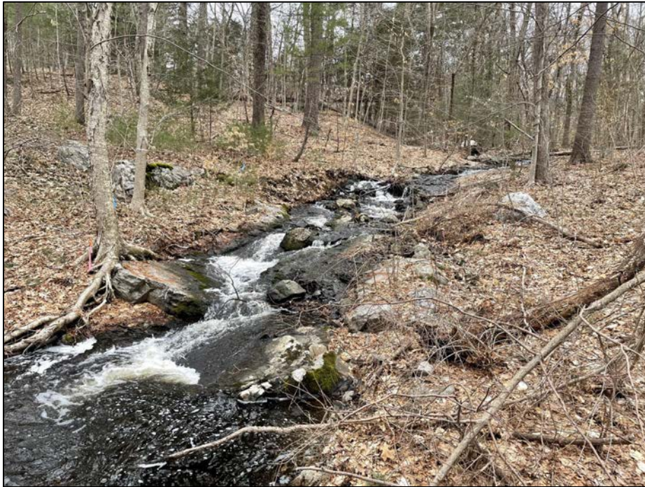
Photo No. 17.: Discharge channel of the spillway from the downstream channel looking upstream. Note the apparent bedrock outcrops throughout.
