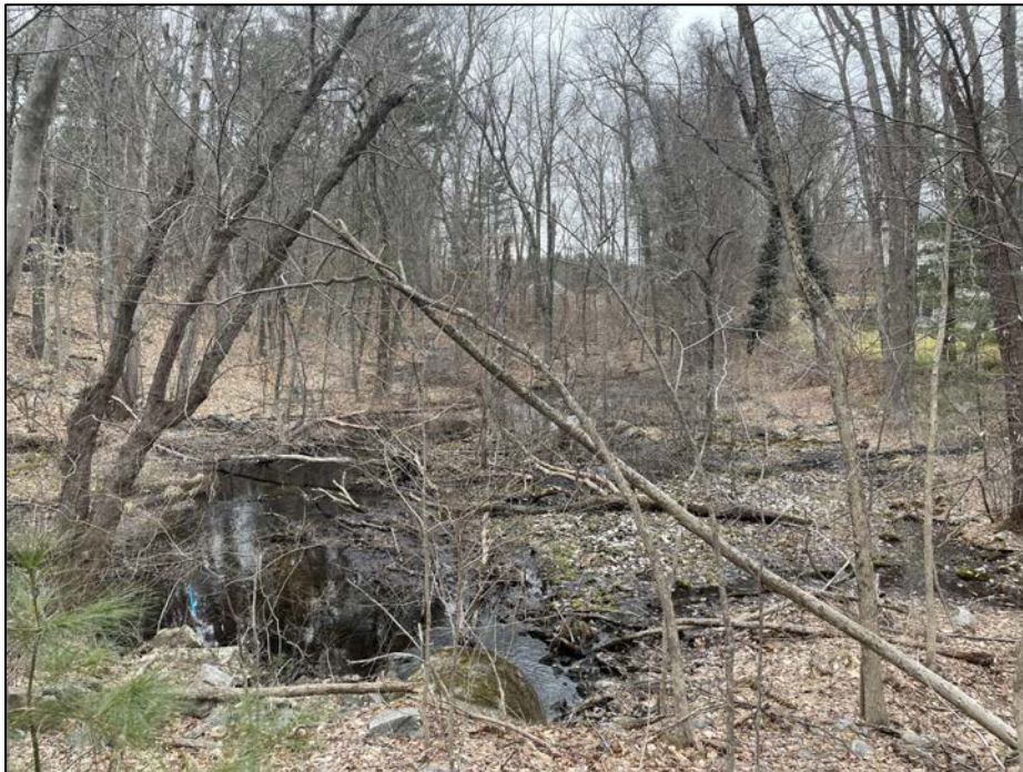
Photo No. 22.: Downstream channel from Woodbridge Road looking upstream.
