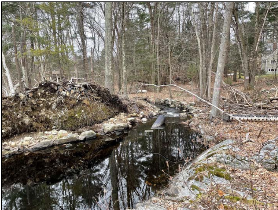
Photo No. 12.: Spillway control section from the approach looking downstream.
