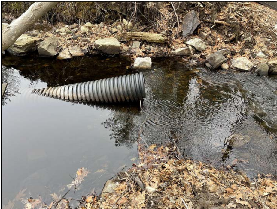
Photo No. 13.: Spillway control section. Note beaver deceiver pipe.
