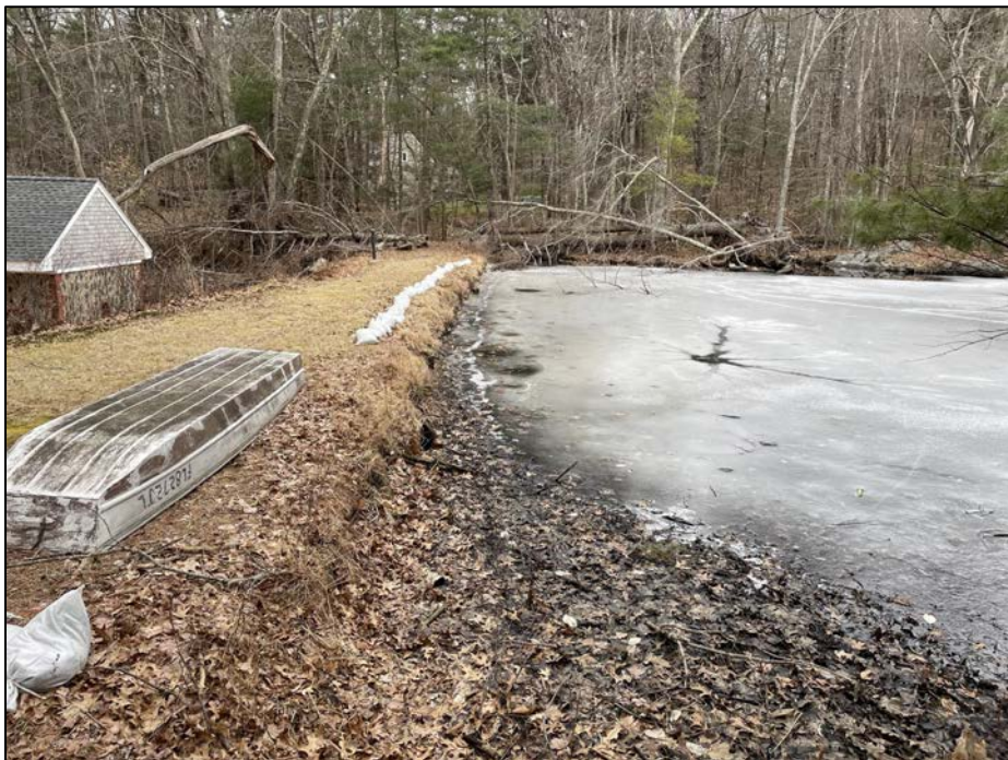
Photo No. 4.: Upstream slope from the left abutment looking right.
