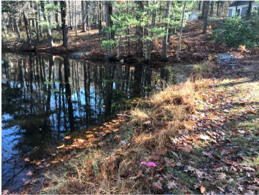
Photo 1: Bank along upstream slope of embankment, consisting of maintained grass slope.
