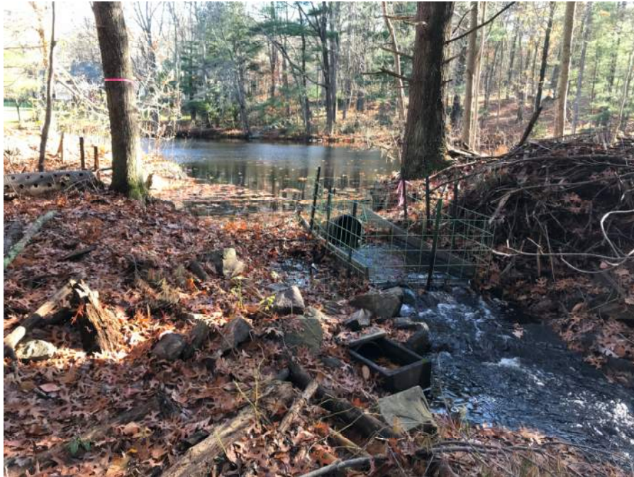
Photo 5: Uncontrolled spillway with beaver control device at right abutment.
