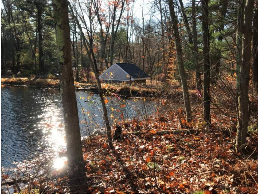
Photo 3: Wooded section of bank at upstream right side of dam, facing southeast toward gatehouse.
